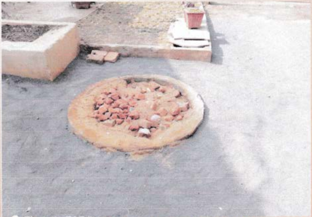
Soak Pit Construction in Campus – For Water Percolation in Groundwater
